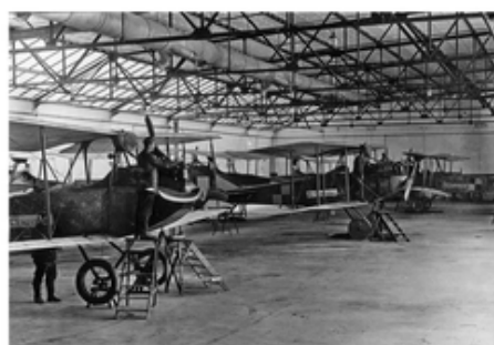
Workshops of the Air Base in Ławica. In the photo there are reconnaissance aircraft - a Rumpler C.Ib No. 124/18 (German No.: 3088/18), a C.I No. 13/... and one other aircraft whose number is not visible, also an Albatros C.Ia No. 118/17 (German No. 15559/17). Photo from the collection of Priest R. Kulczyński SDB
