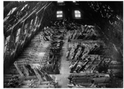
The interior of the aircraft hangar in Winiary near Poznań, filled with airframes. Visible are the fuselages of the following aeroplanes: Albatros B.II, AEG C.IV, AEG N.I and LVG C.V. Photo from the collections of the "Polona" Digital National Library
