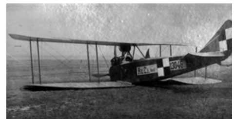
Greater Poland's Rumpler C.I No. 13046/17 after an unfortunate landing. Taken over by the Greater Poland insurgents on 6 January 1919, it was in stock at the Air Base in Ławica, at least till the end of August. Photo from the collections of the "Polona" Digital National Library
